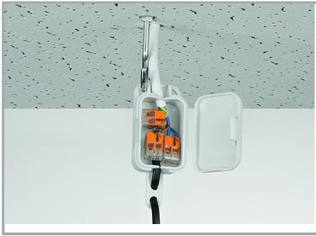
Pendant light connection in a suspended ceiling
