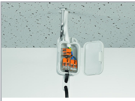
Pendant light connection in a suspended ceiling
